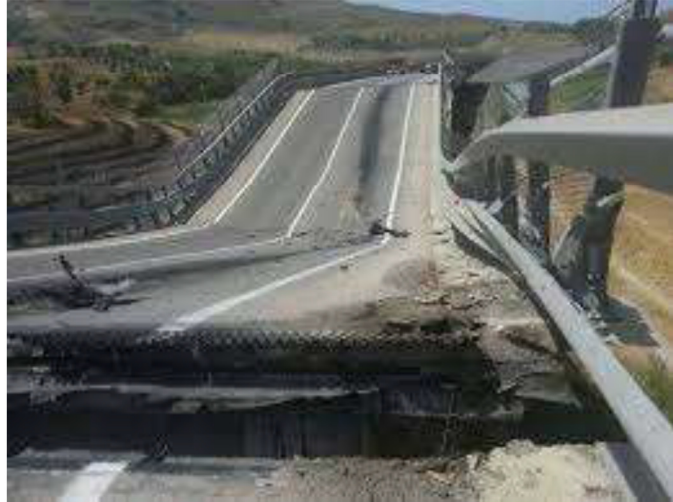
2015 April 10 th , A19 Highway HIMERA VIADUCT between Palermo and Catania
