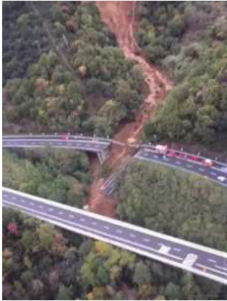
2019 November 24th – A6 Highway MADONNA DEL MONTE VIADUCT close to Savona
