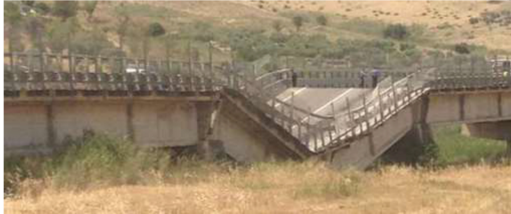
2014 July 7 th , SS626 PETRULLA VIADUCT between Ravanusa e Licata (AG)
